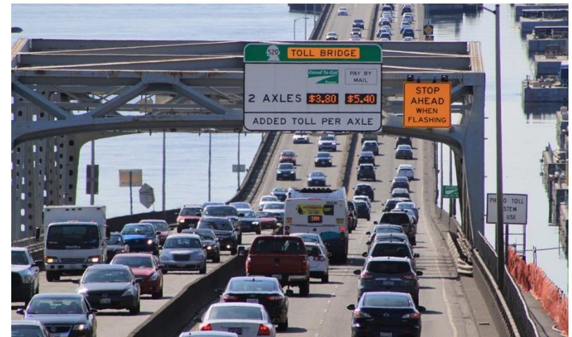
Figure 2: Evergreen Point Floating Bridge (SR 520 Bridge)
