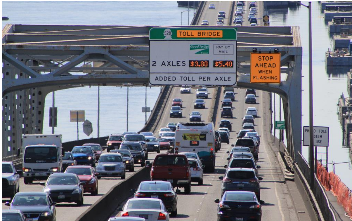
Figure 2: Evergreen Point Floating Bridge (SR 520 Bridge)
